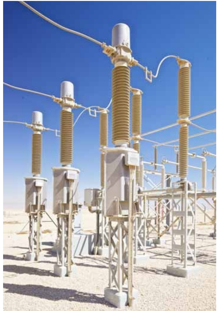
Current transformer IMB 145
